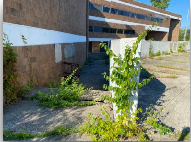
Photo 6: Northeast Corner of Existing Building Facing West Depicting Lower Level.
