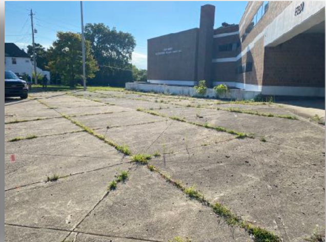
Photo 2: Northwest Portion of the Site Facing East
