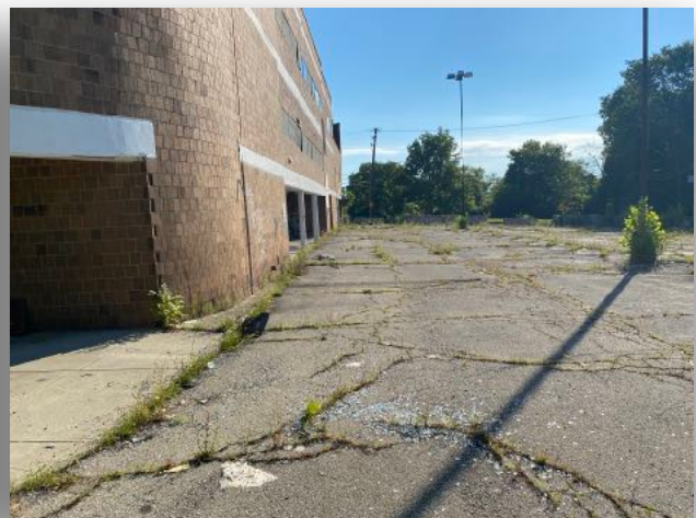
Photo 4: Southwest Corner of Existing Building Facing East.
