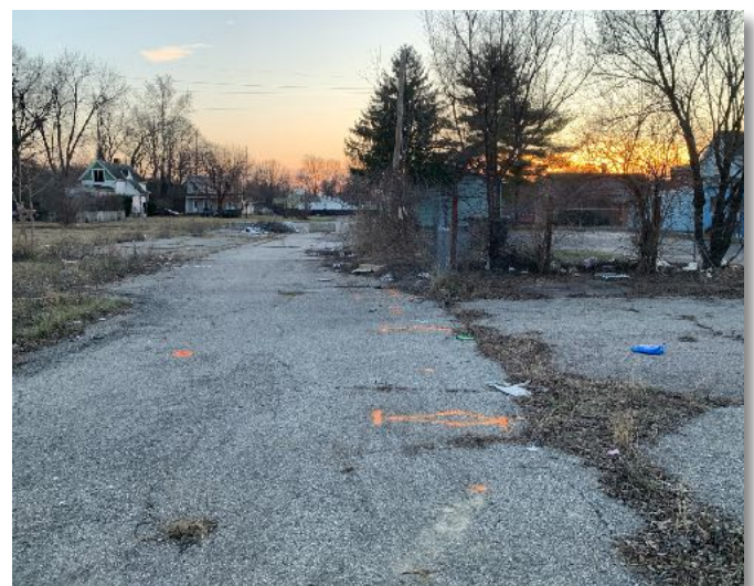
Photo 2: View of Poplar Street and marked underground utilities near center of site
