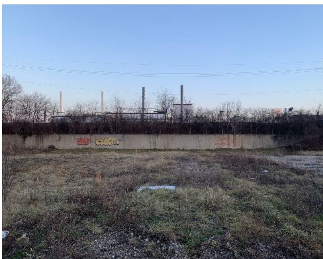
Photo 1: View of existing retaining wall
