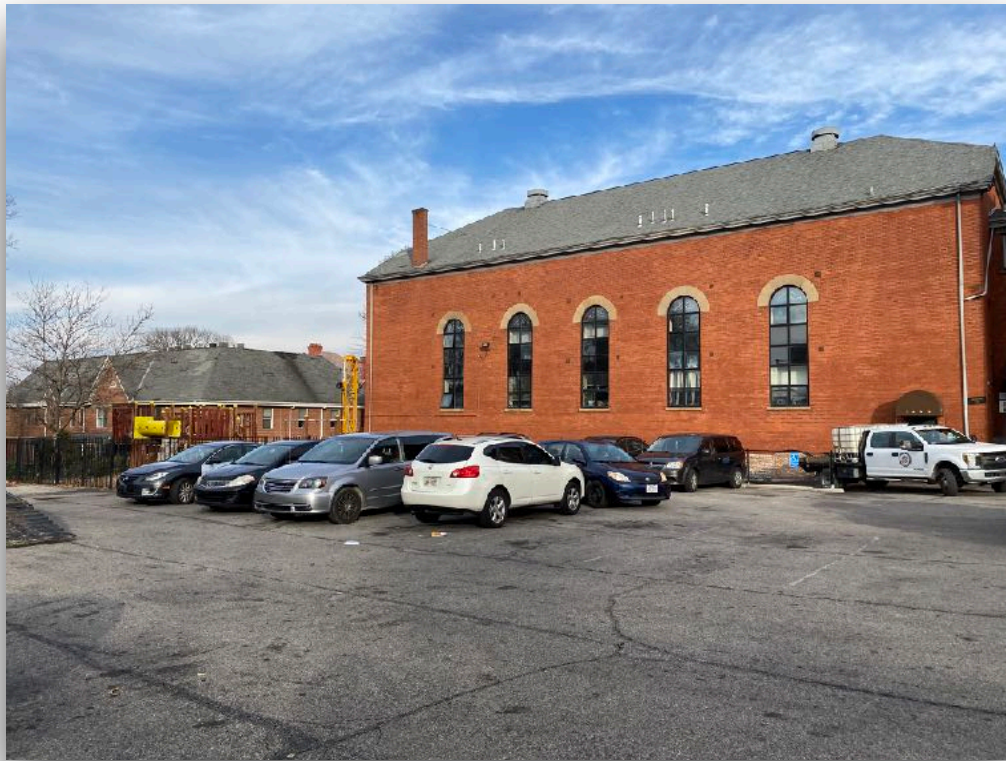
Photograph 2: South end of site facing northwest toward existing building.
