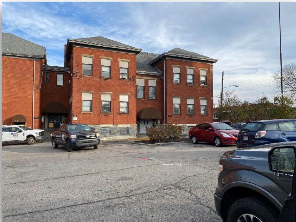
Photograph 1: South end of site facing northeast toward existing building.
