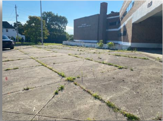
Photo 2: Northwest Portion of the Site Facing East
