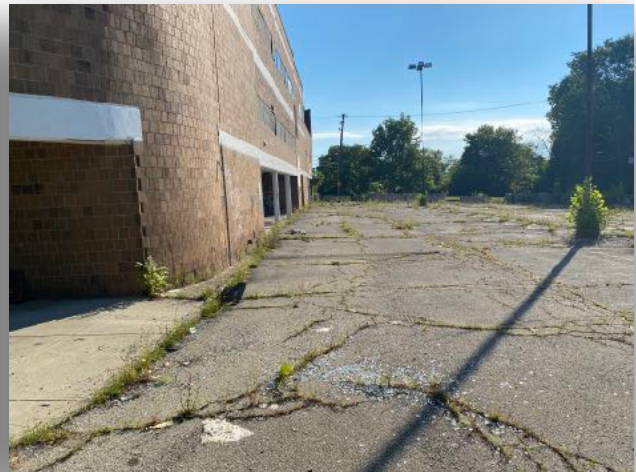
Photo 4: Southwest Corner of Existing Building Facing East.
