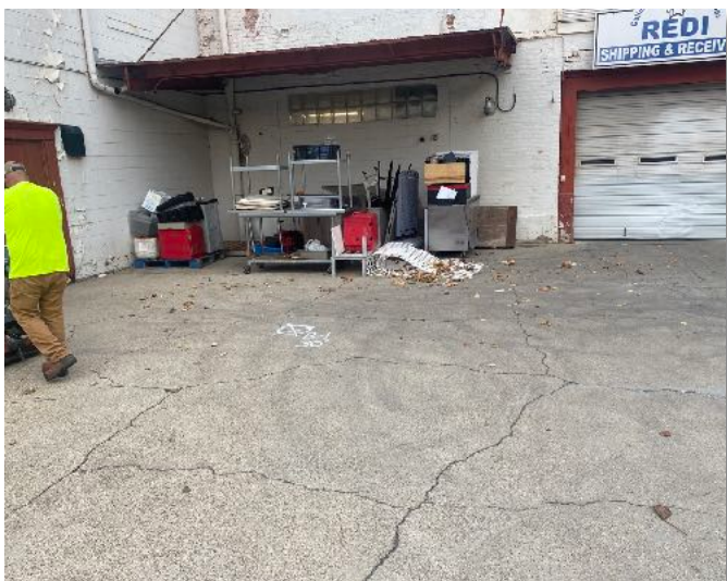
Photo 3: View of existing building and B-1
