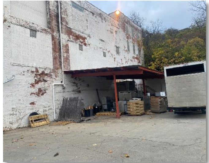
Photo 2: View of existing building.
