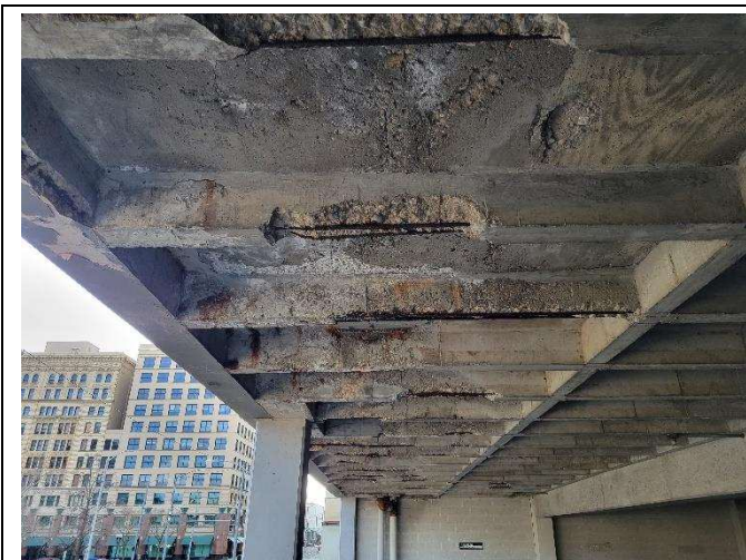
Photo 17 – Joists Pans Replace
