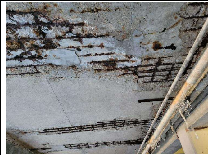
Photo 27 – Replace Flat Slab Section
