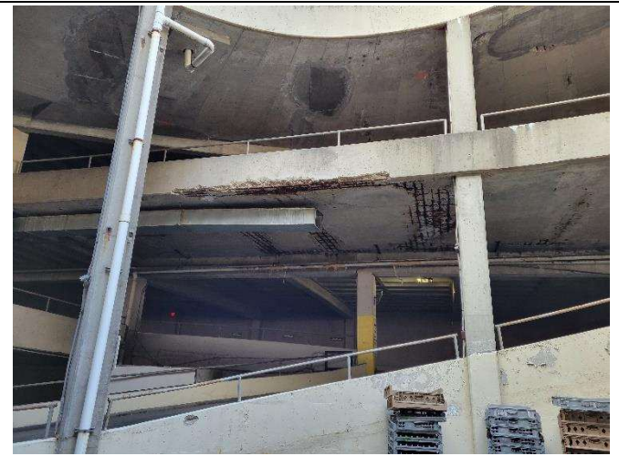
Photo 28 – Replace Flat Slab Spandrel Beam
