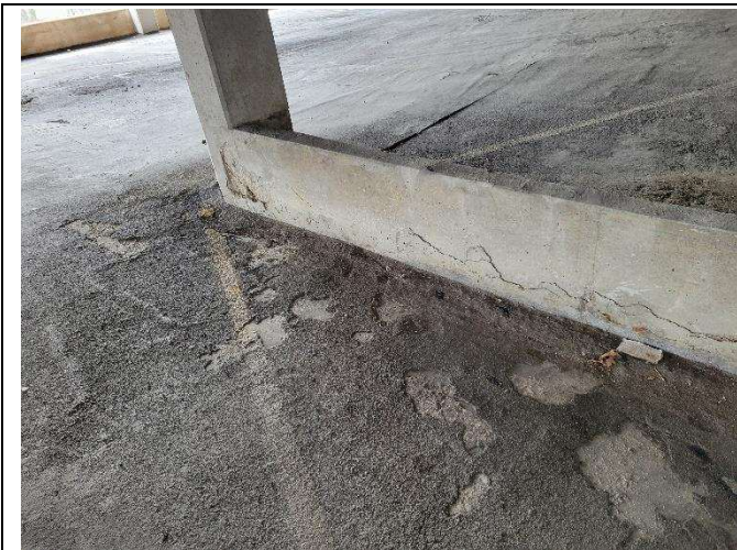
Photo 9 – Divider Wall Topping Repair
