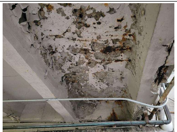
Photo 18 – Pan Deteriorated
