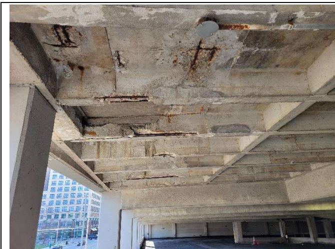
Photo 29 – Replace Section of Bay
