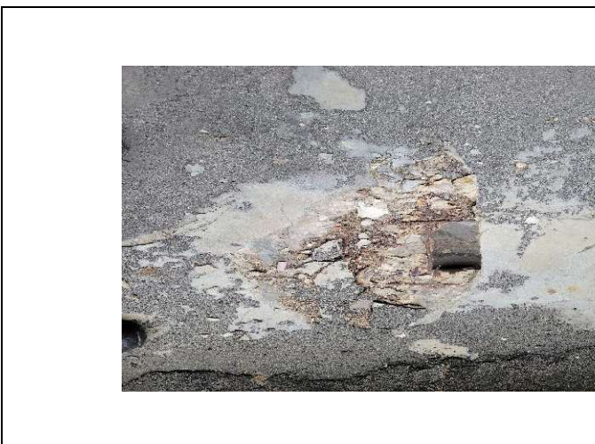
Photo 11 – Holes to be Repaired
