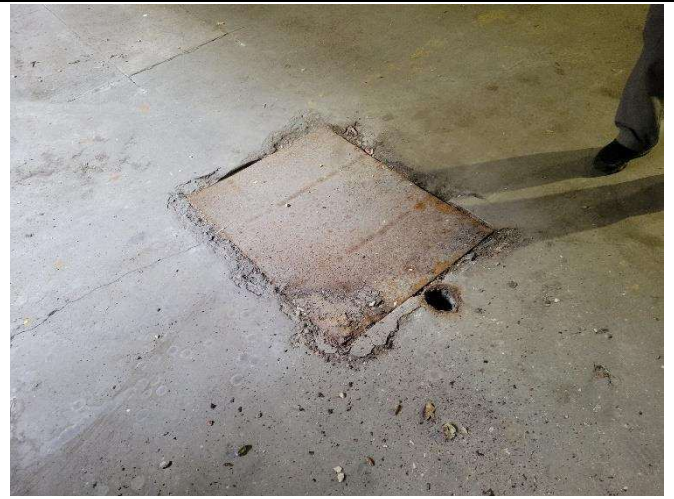
Photo 32 – Slab on Grade Opening Wood Cover
