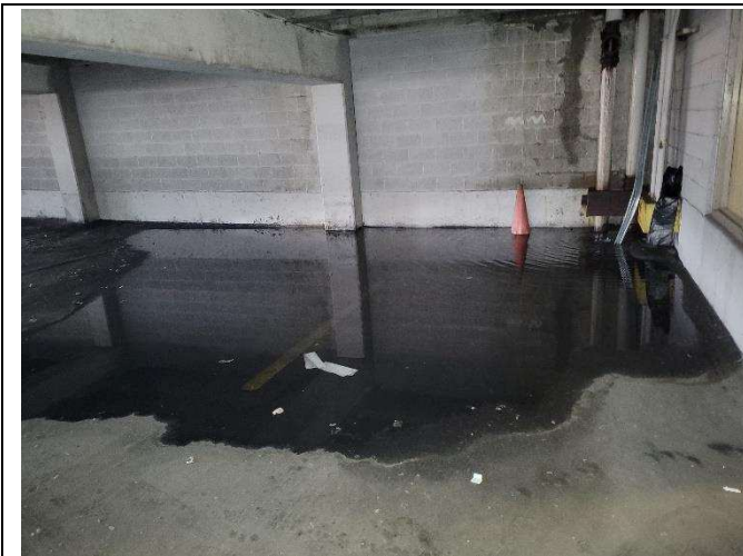
Photo 21 – Ponding at Elevators Wall Damage
