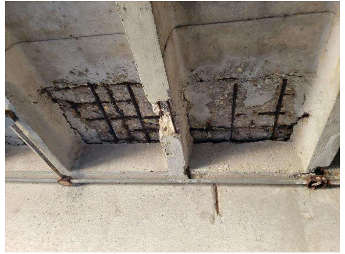
Photo 14 – Joist Pan Wall Repairs
