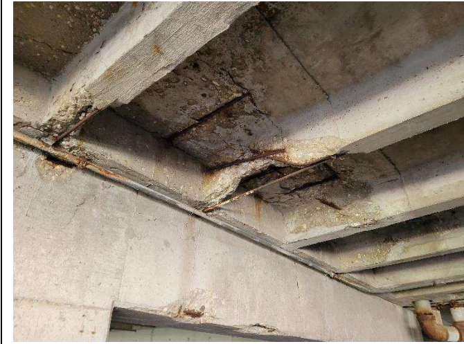
Photo 13 – Joist Pan Beam Repairs
