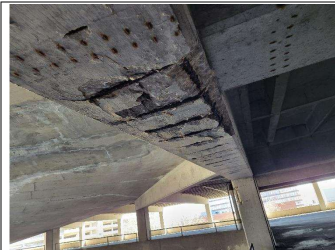
Photo 3 - Beam Ties Bot Bar
