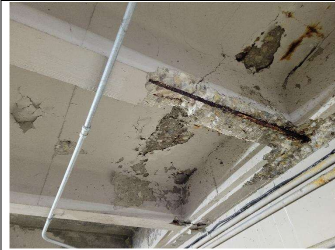
Photo 31 – Shear Crack Add Steel Repair
